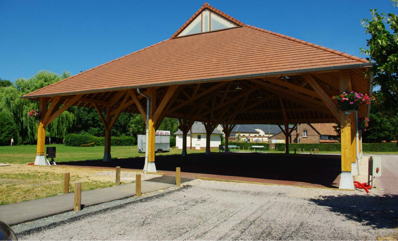
Covered area - Glulam structure with Résix® assembly - Saint Paul (France)
