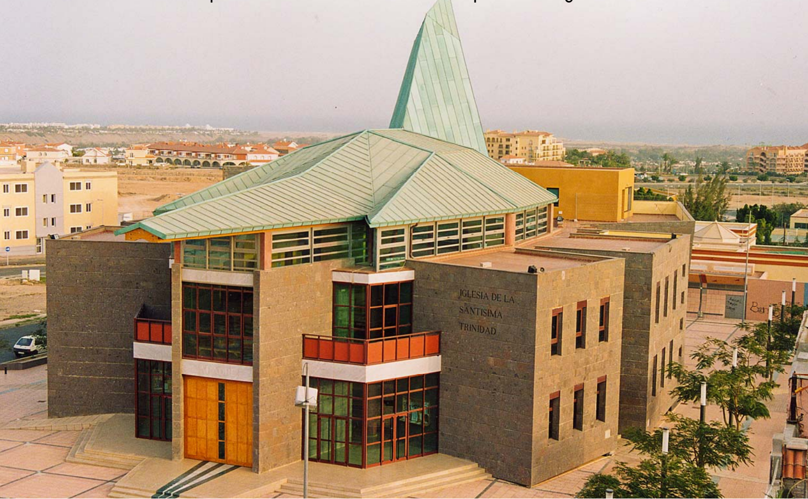
Church in Maspalomas - Glulam structure and Sapisol® roofing - Gran Canaria
